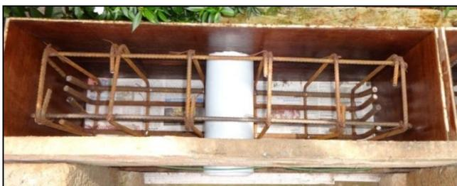
Fig. 2. Shuttering and placing of reinforcement cage for deep beam
