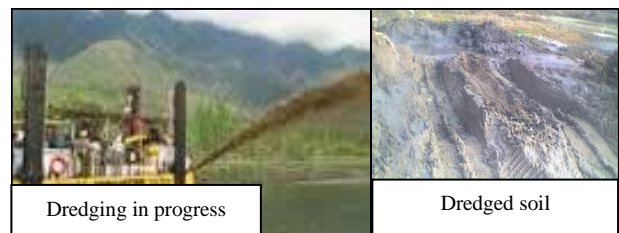
Fig. 1. Dredging of Dal Lake in progress and accumulation of dredged Soil along Lake Shores
