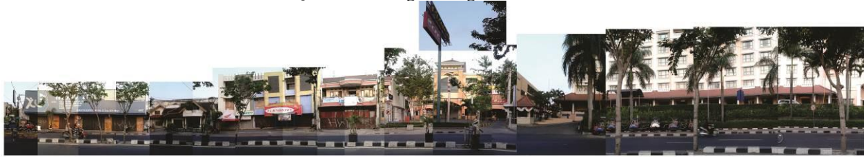
Fig. 12. Montage of Segment IV-West
