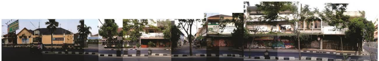
Fig. 6. Montage of Segment I-West
