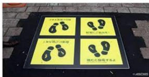
Fig. 5 : Piezoelectric Tiles near Tokyo Railway Station
