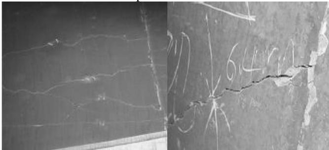
Figure 1 lining crack of a tunnel (Mined out area in the low of the tunnel)
