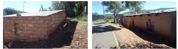
Fig.5. Images showing buildings used as retaining walls
