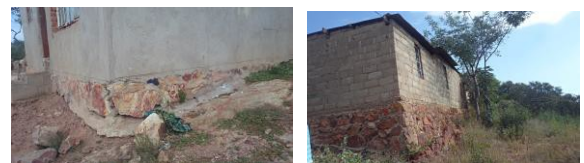
Fig.7. Image showing rocks used as foundation footing
