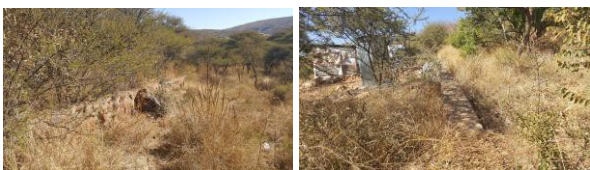
Fig.2. Images showing storm water retaining wall
