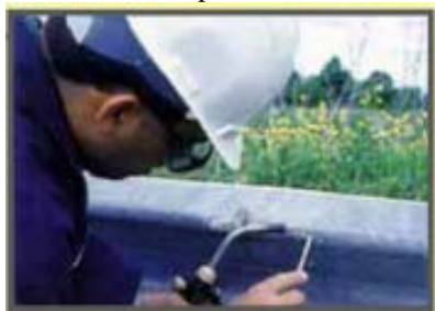
Figure 4: Zinc-Based Solder Technique
