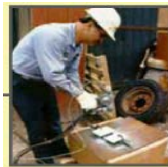
Figure 6: Zinc – Spray (Metallizing)
